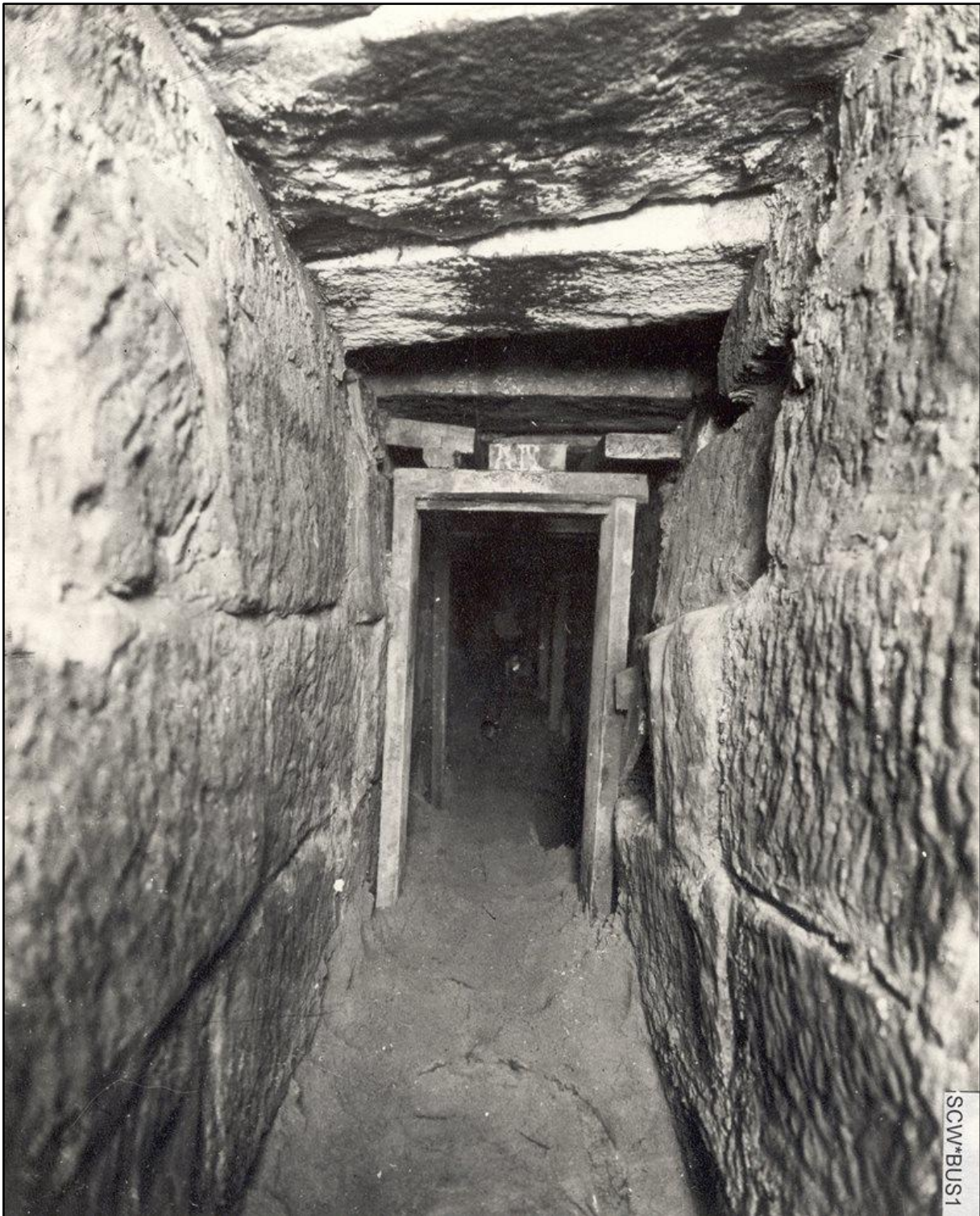
Figure 8: Busby's Bore at the intersection of College and Liverpool Streets, constructed with stone masonry lining. Source: Sydney Water Archives. Note: This type of construction was not used in the construction of the Busbys Bore Spur
