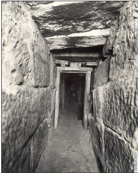
Figure 7: Busby's Bore at the intersection of College and Liverpool Streets, constructed with stone masonry lining. Source: Sydney Water Archives. Note: This type of construction was not used in the construction of the Busby's Bore Spur.
