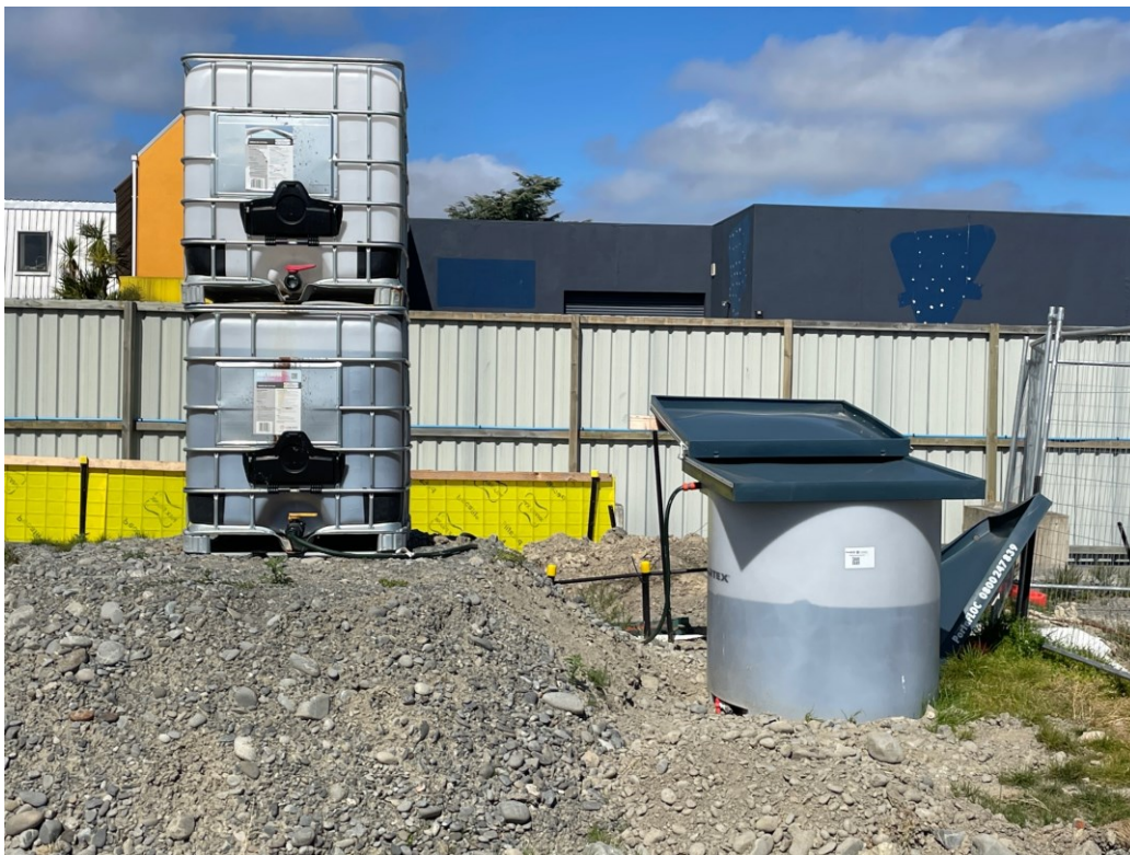
Examples of auto-dosing systems on BESIX Watpac sites
